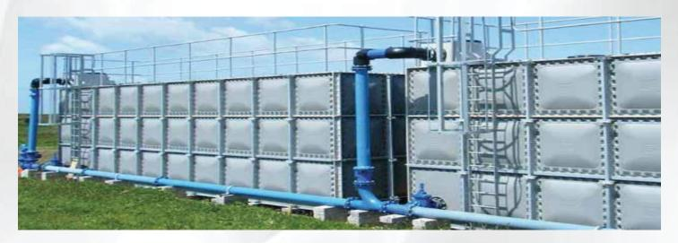
GRP panel type water tanks are a type of water storage system constructed using strong and durable Glass Reinforced Plastic panels. These tanks are designed to store water efficiently, making it readily available whenever needed. Whether for residential, commercial, or industrial use, GRP panel type water tanks provide an effective and reliable solution for water storage.
