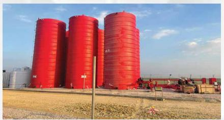
Fire water storage tanks are used to provide facilities with potential fire hazards, directly controlling the amount of water necessary to ensure that fires can be put out in a timely manner and appropriate water resources are available
